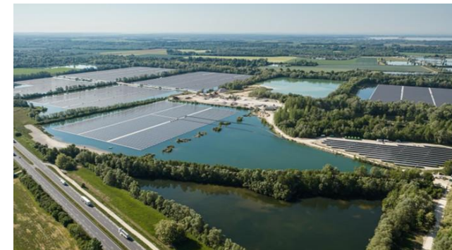
France, Perthes, 2025, 72MWp Q Energy, Ciel&Terre
