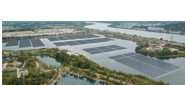
France, Piolenc, 2019, 17MWp + Extension of 5 MWp in 2022 Akua, Ciel&Terre
