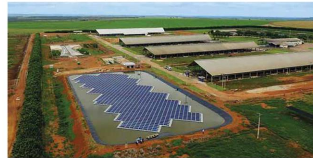
FIGURE 3.4. FPV system (of 305 kWp capacity) in Goiás, Brazil
