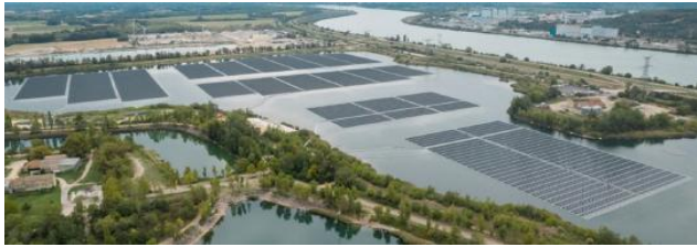
France, Piolenc, 2019, 17MWp + Extension of 5 MWp in 2022 Akua, Ciel&Terre
